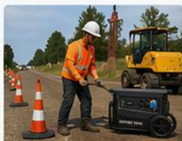
ROAD WORKS & CONSTRUCTION
